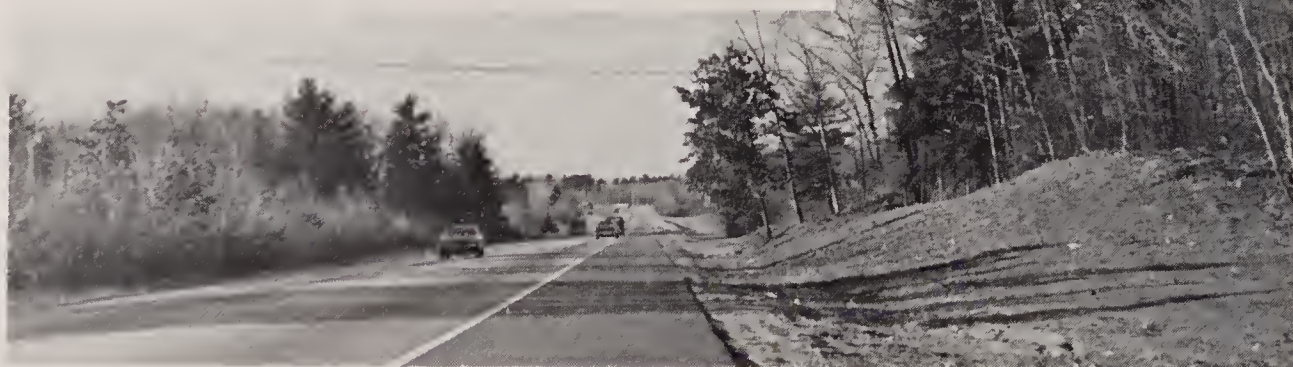
Route 125 was extended into Wilmington
